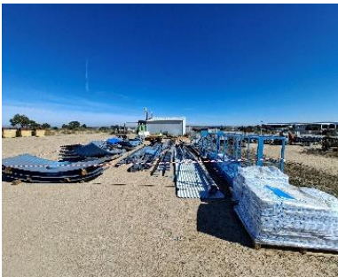
Recepción material deposito PCI
